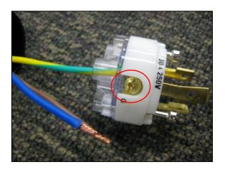
8. Fasten the cover of the plug by tightening the screws.
